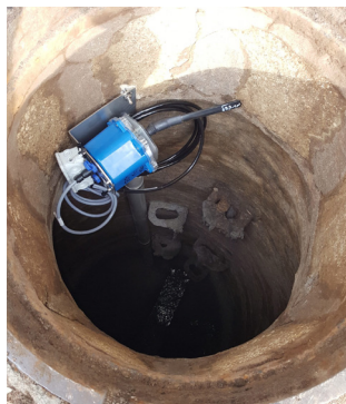
SEWAGE PIT LEVEL MONITORING
